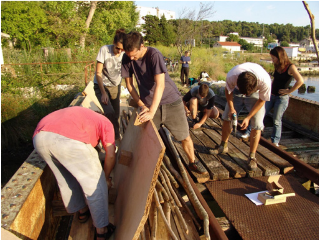
Reconstruction of the Bridge to Valelunga
